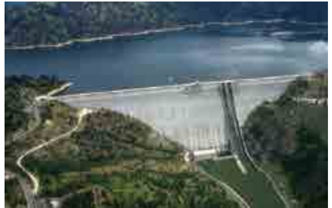
Dworshak Dam, Idaho
